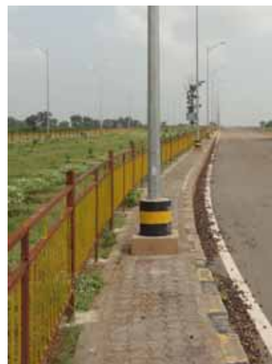
Figure 3: Lamp posts on footpath (photo by WB mission)
